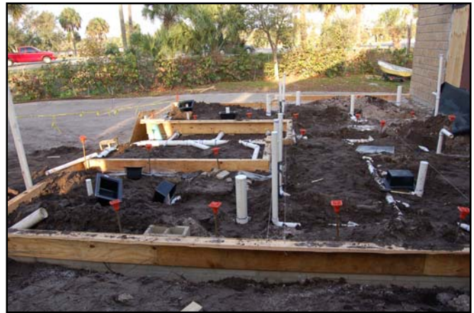
New restrooms and shower area before (above) and after (below) the concrete slab was poured.
