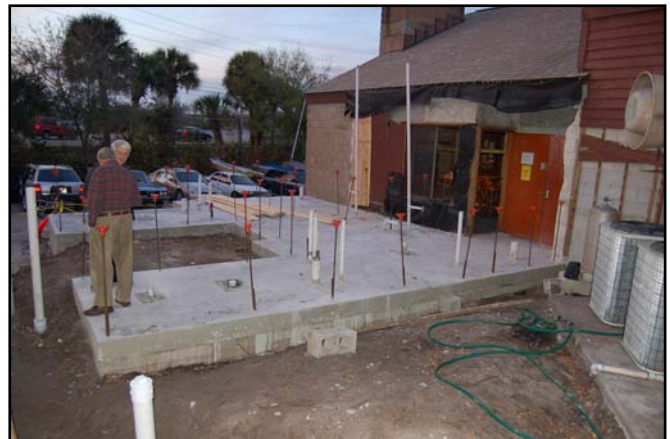
New restrooms and shower area before (above) and after (below) the concrete slab was poured.
